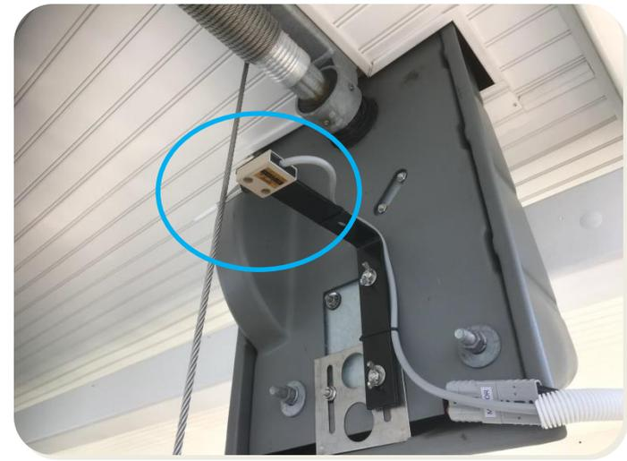
**IMPORTANT:** Install the limit switch in a location that will trip when the desired amount of cable has been spooled.
